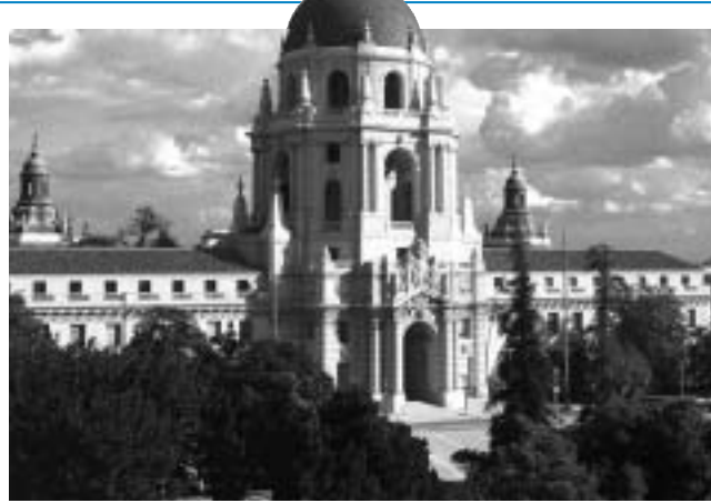
For nearly 80 years, residents, architects and preservationists have stood in awe of Pasadena City Hall's magnificence. The dome of City Hall is commanding yet graceful. The massive circular structure rises six stories.
